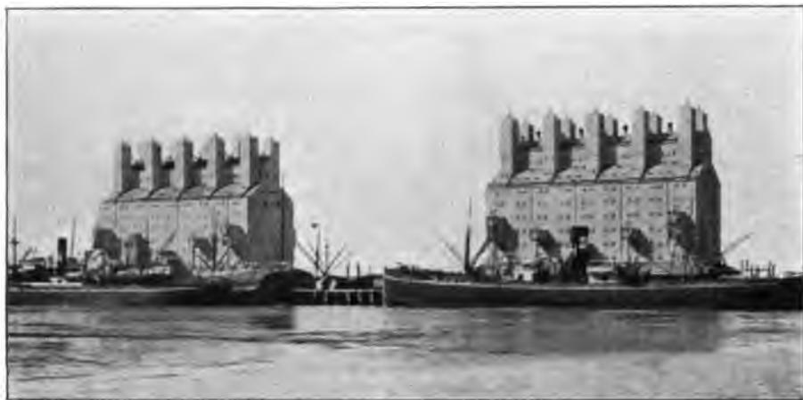
Grain Elevators, Bahia Blanca, Argentina
